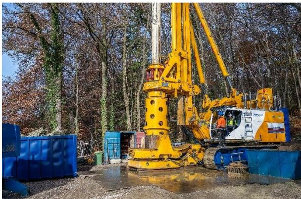
(4) The particular challenge on this project: precise work in varying soil strata including rock, down to an unparalleled depth of 160 m.
