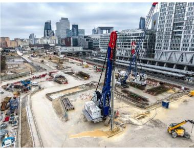
(1) By 2027, the BAUER BCS 185 power pack will be used at several new stations on Line 15 of the Paris metro to carry out diaphragm wall works.
