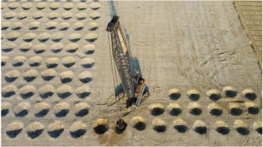
(2) After the initial phase, to ensure compaction over the entire area, the points between the individual craters are worked on with the pounders during the second phase.
