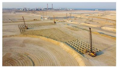
(1) Soil compaction for the Sabah Al Ahmad Sea City construction project – a total of six BAUER MC duty-cycle cranes are being used in Kuwait under extreme conditions.
