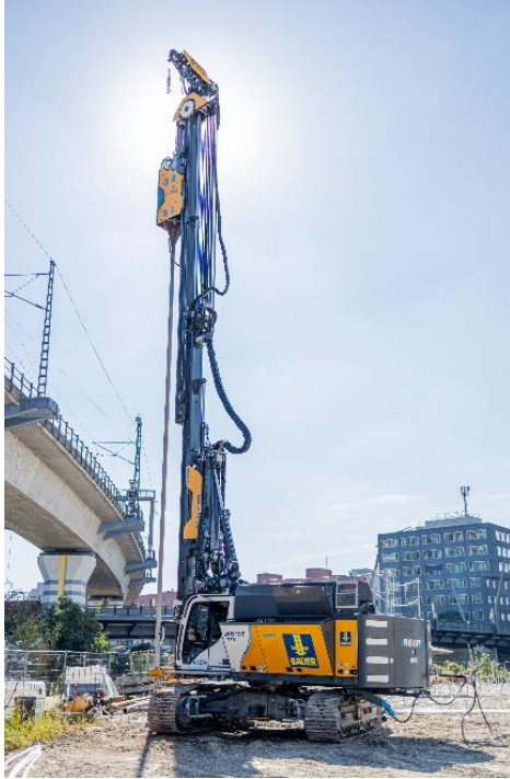
(1) First deployment of eRG 19 T hybrid from RTG Rammtechnik in Berlin.
