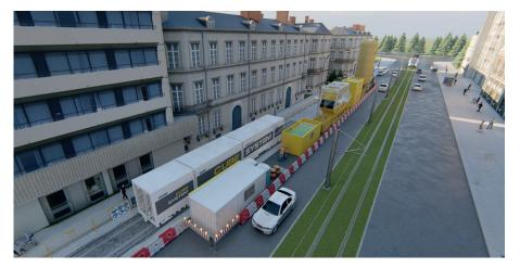
at sites with limited space or requirements to cause as little impact on traffic as possible. The modular design of the slurry handling equipment allows individual arrangements to comply with the specific needs.
