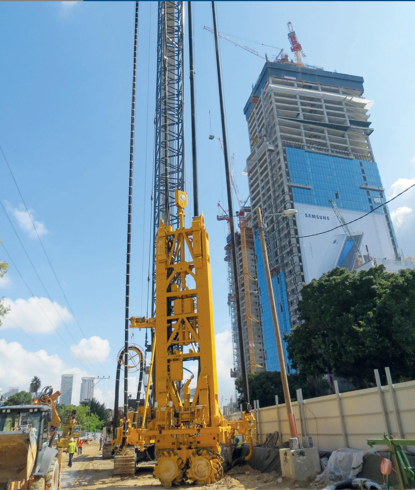
A continuous wall is constructed by a series of independent rectangular panels. The open trench is supported and stabilized during excavation by a thixotropic slurry. Subsequently, a reinforcement cage is lowered into the open trench and concrete or self-hardening sealing material (plastic concrete) is placed into the trench from the bottom up using tremie pipes.
