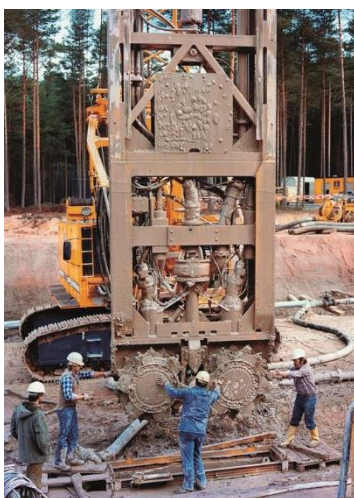
(1) The first Bauer cutter at work sealing the Brombach reservoir in 1985.
