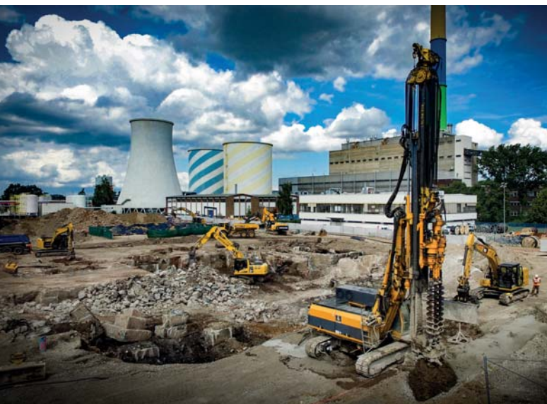
Chemnitz, Germany Cleanup works at power plant
