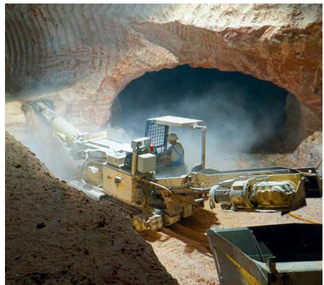
Bleicherode, Germany Conventional drifting with a selective road header
