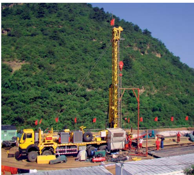
ShanXi, China Coal bed methane drilling
