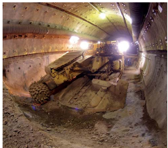
Waste Disposal Konrad, Germany Removal work
