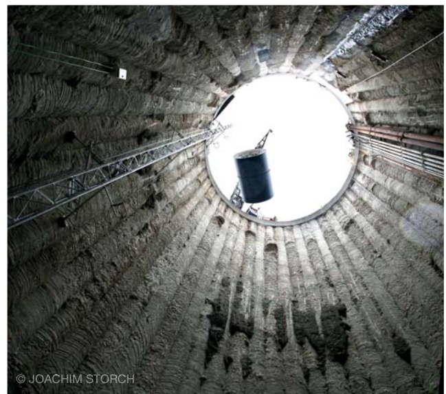
Frankfurt, Germany Construction of vertical shaft with secant pile wall
