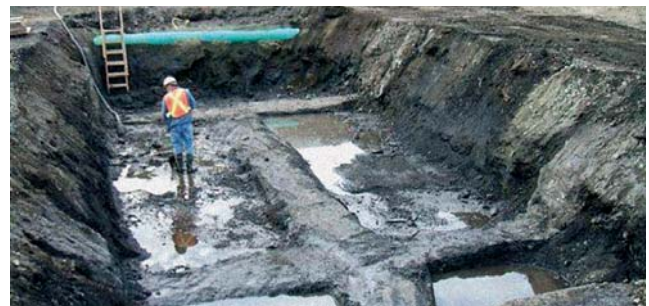
Vancouver, Canada Soil stabilization with soil mixing web-structure
