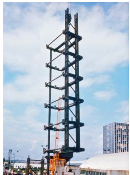
Shaft Sondershausen, Germany Working platform with 6 floors
