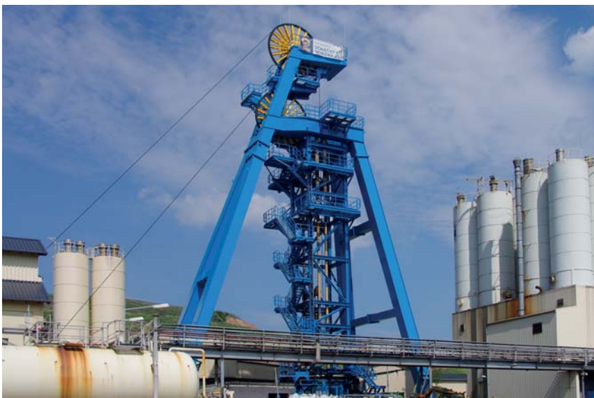
Shaft Sondershausen, Germany Manufacturing and installation of new head frame
