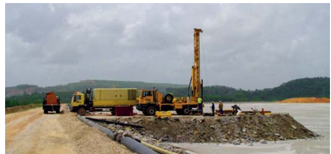
Gold mine, Ghana Drilling of monitoring holes on tailings dam
