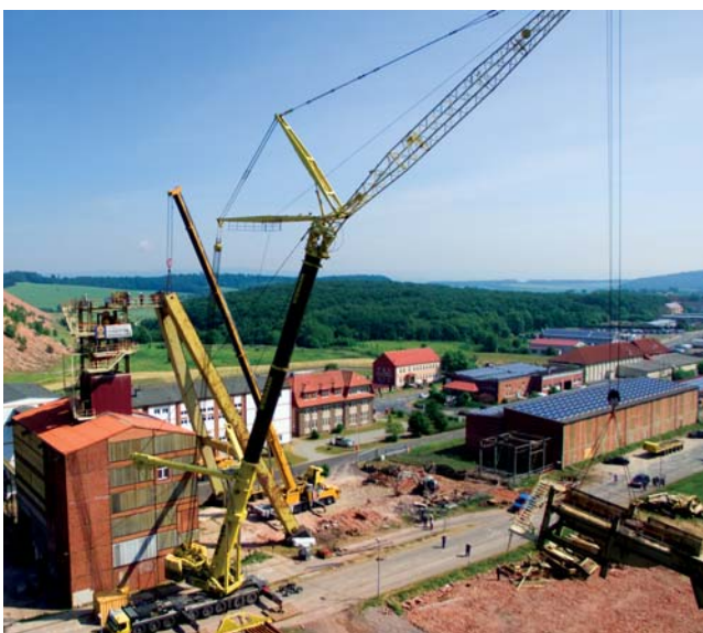
Bischofferode, Germany Dismantling of head frame system
