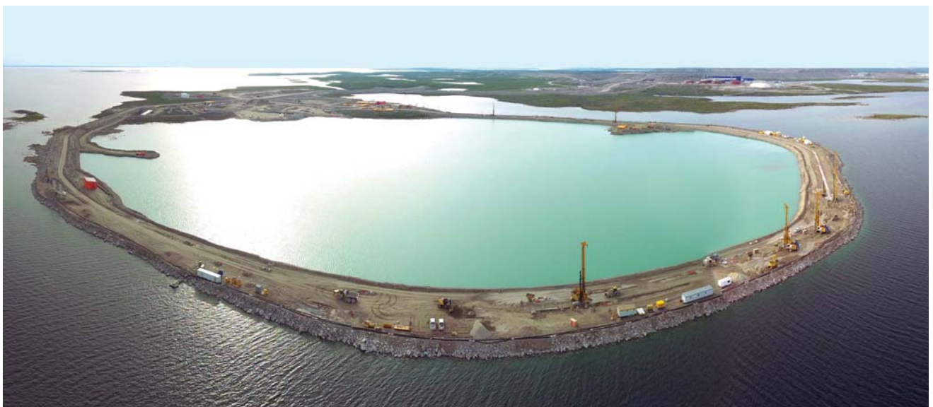
Diavik Diamond Mine, Northwest Territories, Canada Creation of a 26 m deep cut-off wall for the 2.2 km A21 dike
