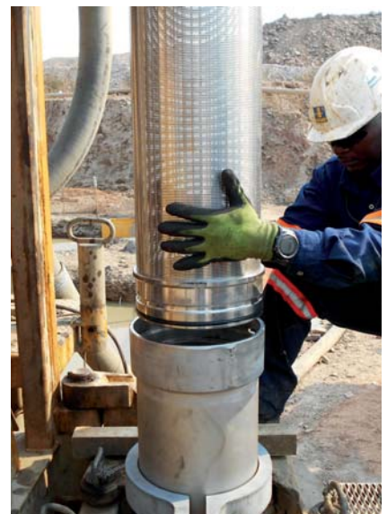
Copper mine, DRC Installation of 16" GWE screens
