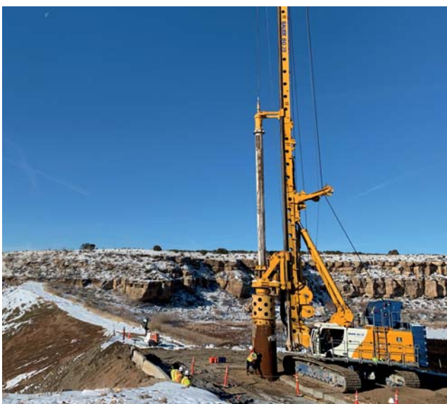
Teller Dam, Colorado, USA Remediation works to intercept seepage and erosion
