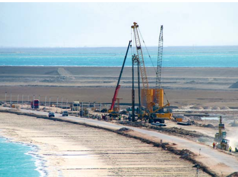
Potash production, Jordan Dike remediation works with 4.2 km long cut-off wall
