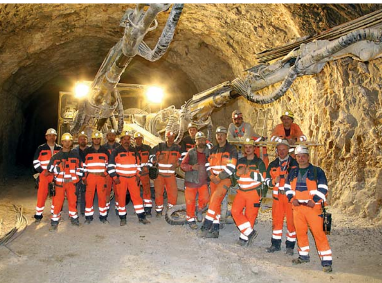
Mähringer Berg, Ulm, Germany Work for a new underground limestone mine
