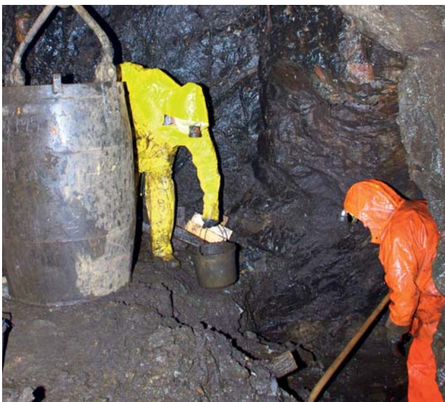
Rothschönberger Mine, Germany Getting in trim of light hole
