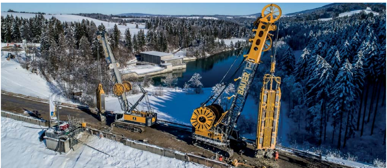
Rosshaupten Dam, Germany Cut-off wall installation with cutter and grab
