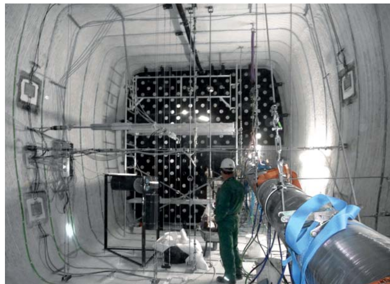
Morsleben, Germany Erection of a sealing structure in rock salt
