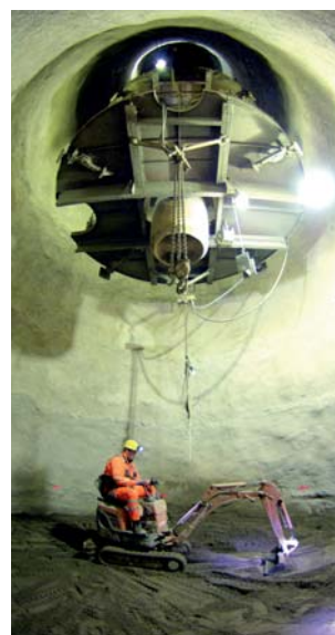
Bischofferode, Germany Installation of shaft sealing
