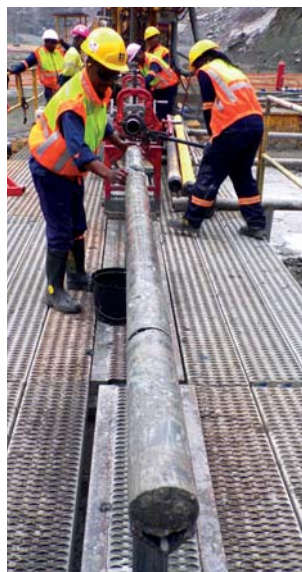
Jwaneng Diamond Mine, Botswana Recovery of 5 ½" core
