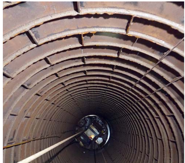
Shaft Lohra Tubbing shaft
