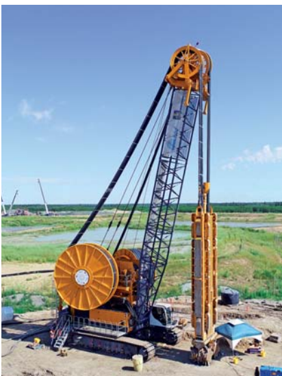
Cutter mining from surface level, Canada
