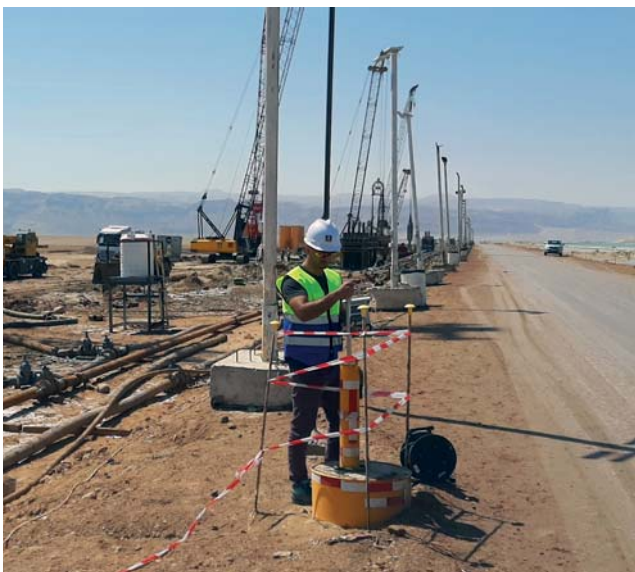
Potash production, Jordan Installation of dike monitoring device
